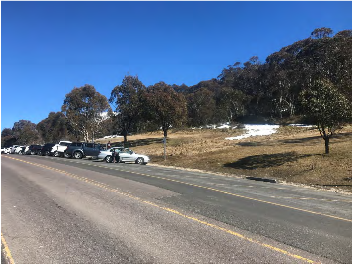
Photo 5: The location of the off ramp in the northern parts of the proposed car park.
